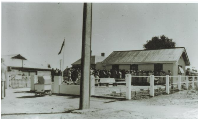
The official opening of the Auburn RSL Clubrooms. The building to the left was the newly established workshop of S.P. Stephens (now part of Beckers IGA). In the background the house is now the French family home. (The Mess Hut was the Male and Female Mess Hut shown in the August 2017 issue of the Auburn Express.) Photo National Trust – Overton collection
